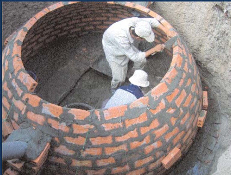
Building a biogas digester in Vietnam ALL IMAGES DW
